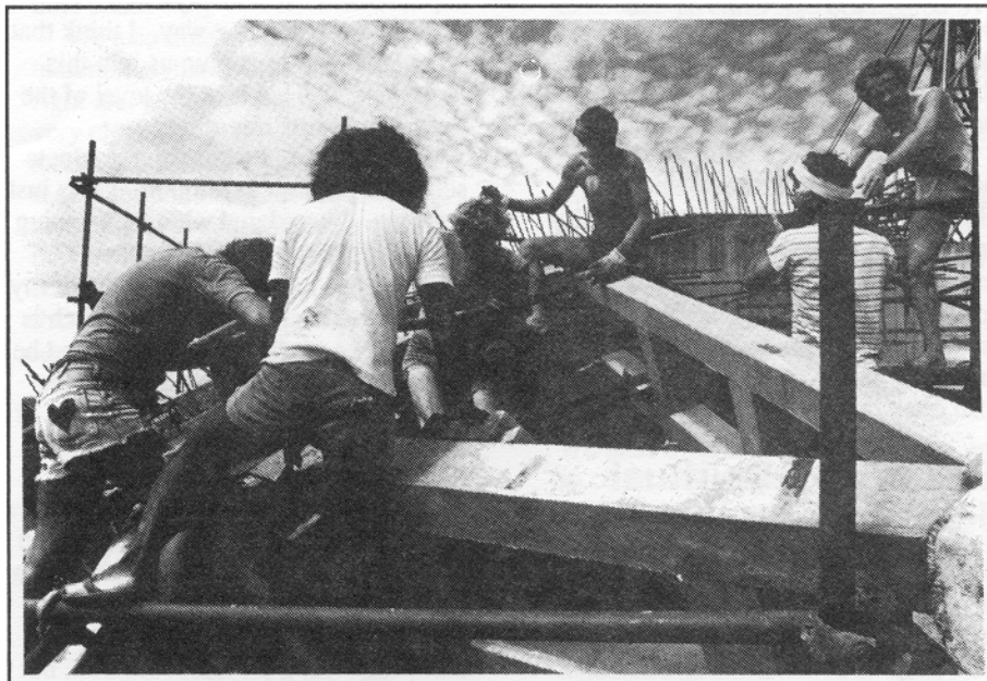
On top of Matrimandir
